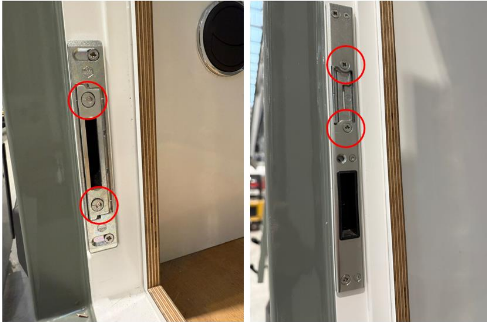
Figure 2: Door Adjustment
